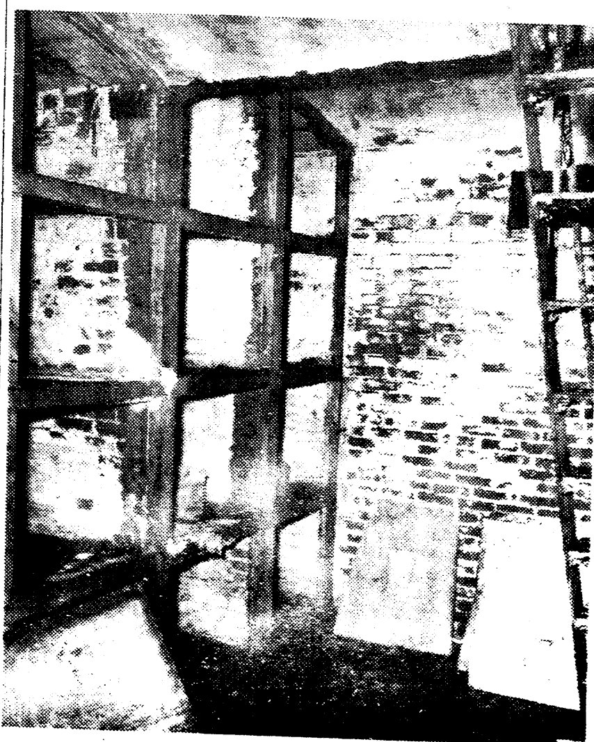
The crypts (lining the left wall) formerly held bodies of dead Mother Superiors. The bodies were removed when the Manhattanville College of the Sacred Heart left the area. On the lower left part of the picture is the slab of stone that was removed by the Observation Post reporter.
