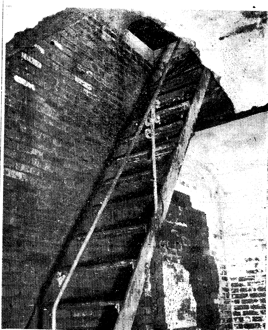
OP Photos by Bourgun This rusty ladder leads to the catacomb. The first few steps are broken. On the wall in back of the ladder a hole reveals the absence of a religious plaque.
